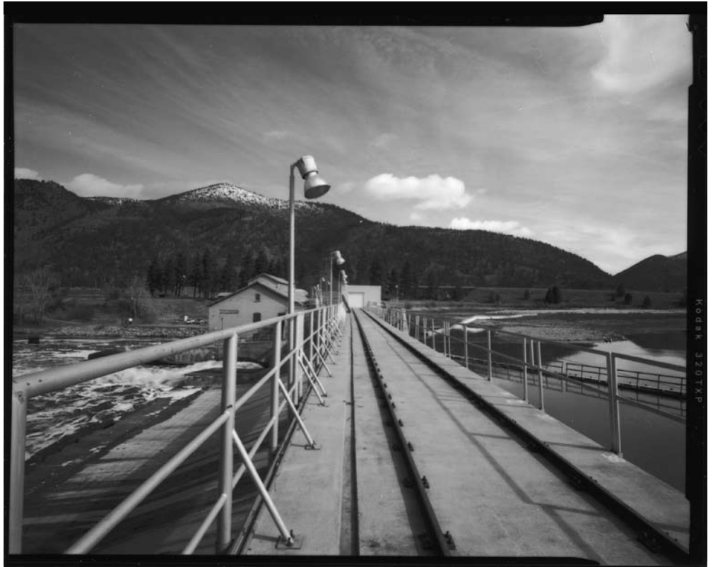
Documentary photos of the interior and exterior of Milltown Dam by Kristi Hagar | Courtesy of NorthWestern Energy
